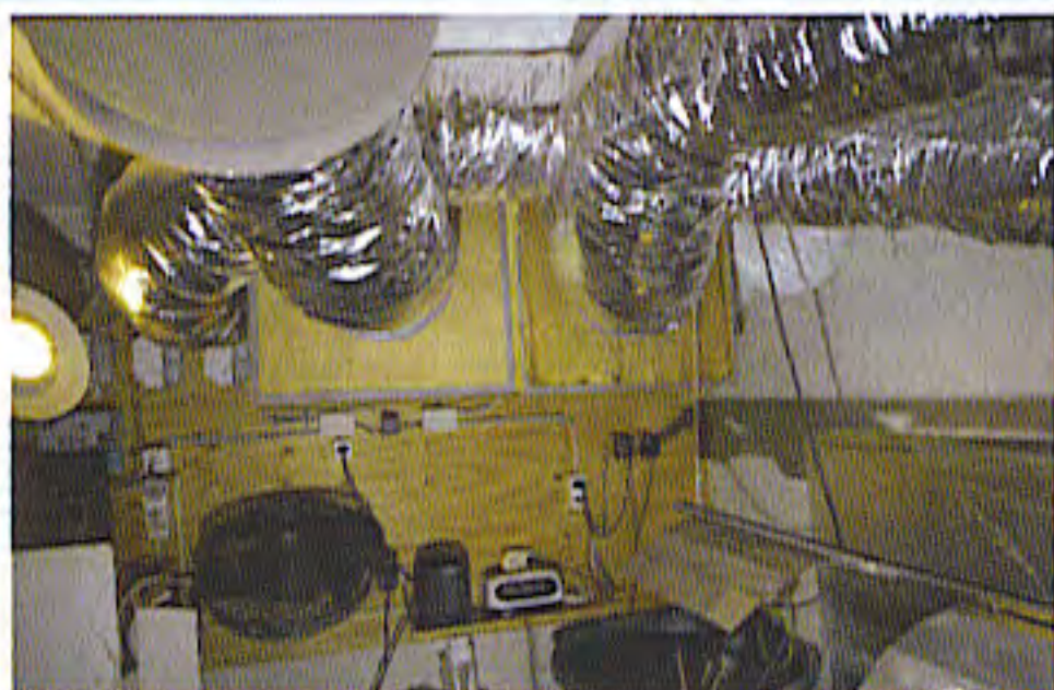
This grower uses insulated ducting to dampen noise and vibrations caused by moving air.
