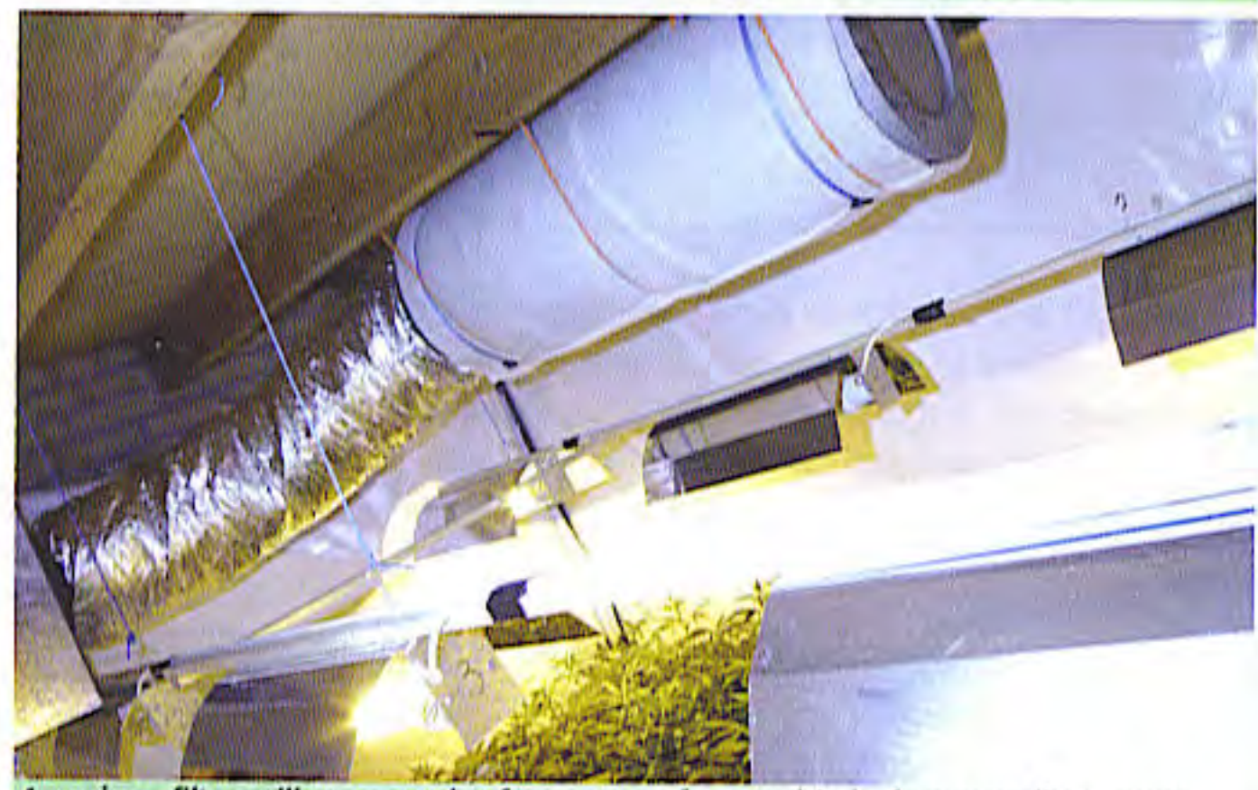
A carbon filter will remove the fragrance of cannabis before expelling grow room air.
